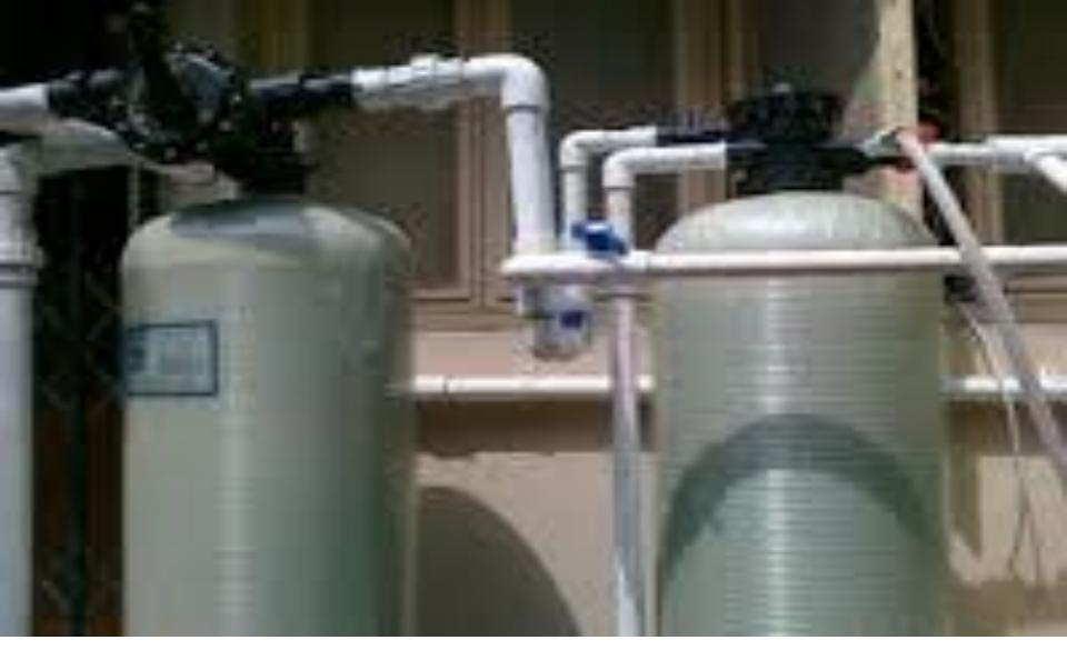
Activated CARBON filter on your pool water make up line. Remove chloramines from city water.
